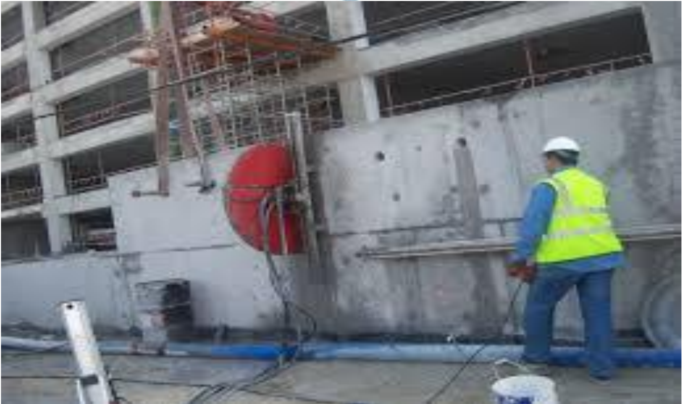
Fig. Wall (Track) Sawing
