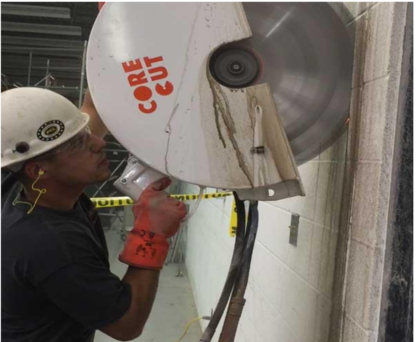
Fig. Core cutting
