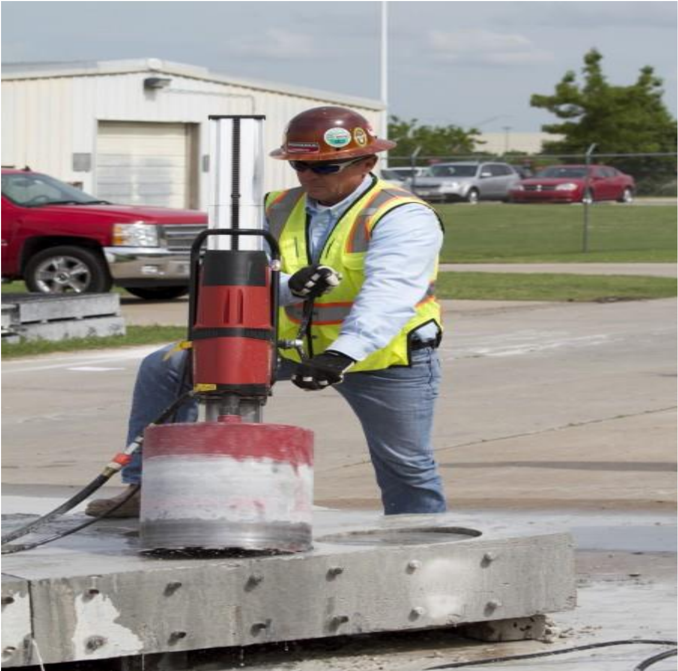
Fig. 1 concrete Drilling cored ho
