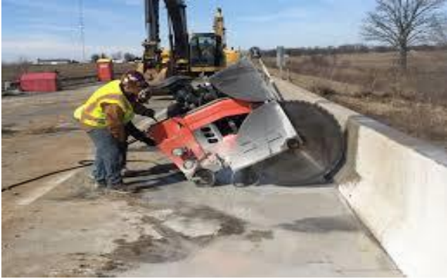
Fig.1concret sawing
