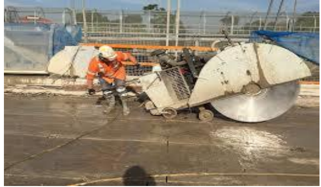
Fig. concrete sawing
