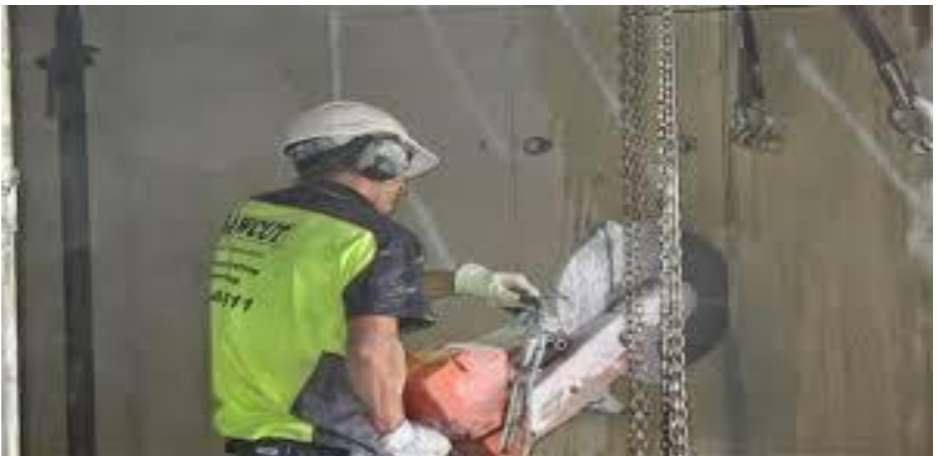
Fig. Wall (Track) Sawing
