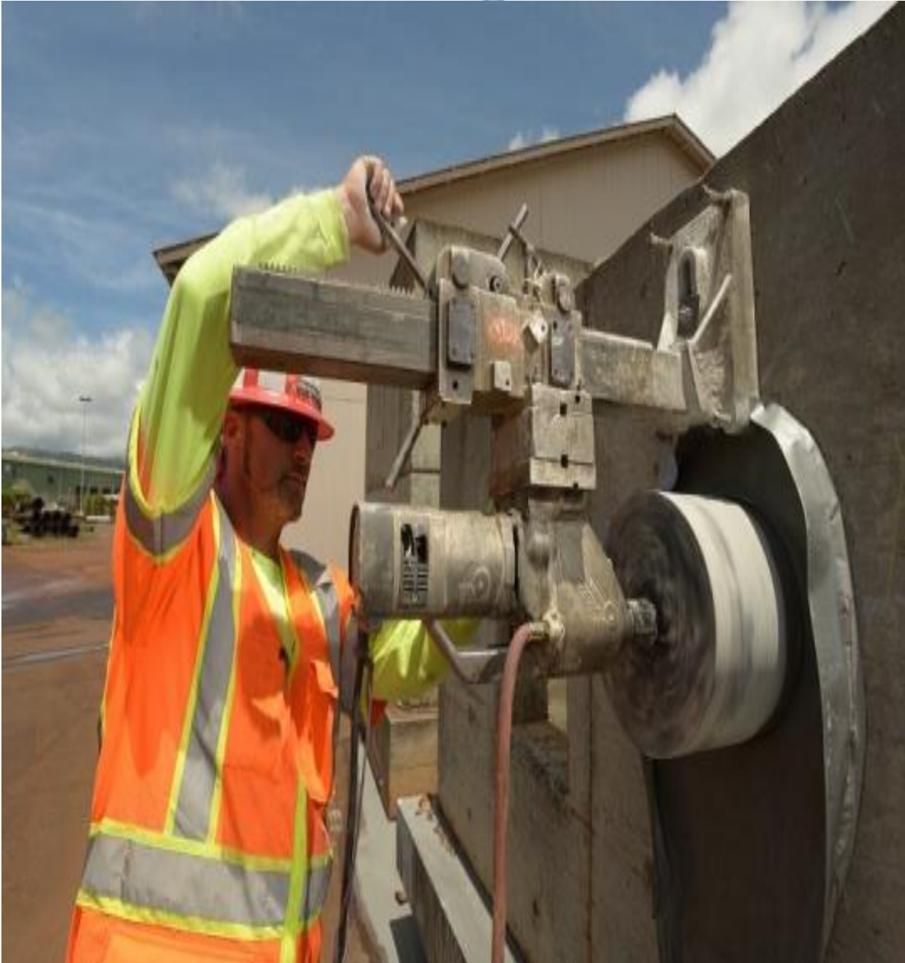
Fig. 1 concrete Drilling cored ho
