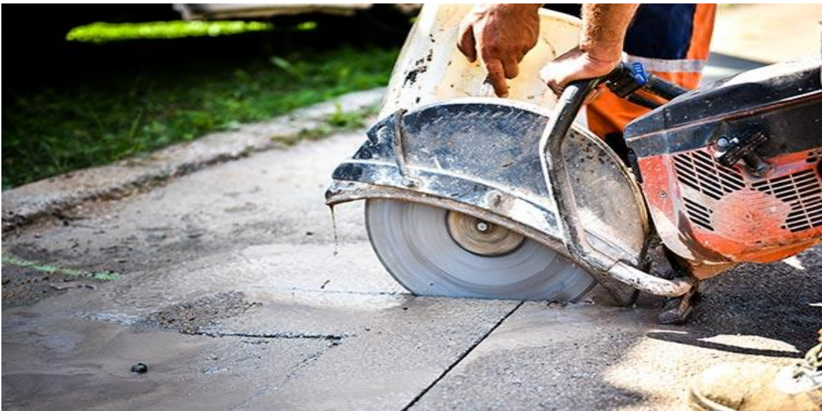
Fig. concrete Cutting
